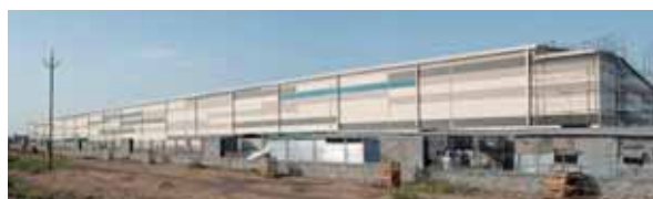
Ferrero Social Enterprise - India (Baramati/Pune, Maharashtra)
